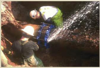
Water Operations crew members repair a leak on an 18-inch water main on Ninth Avenue.
