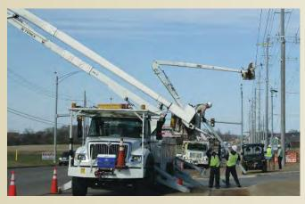
Electric crews are currently working along County Line Road preparing delivery lines for the 46kV portion of the new substation built to feed from TVA's County Line Delivery Point. The 12 kV portion of the substation is already online.
