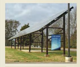
Huntsville Botanical Gardens became the site of a new solar-powered generation exhibit during FY2012. The solar panels have a 23-kilowatt capacity and can generate about 30,000 kilowatt-hours of electricity each year.
